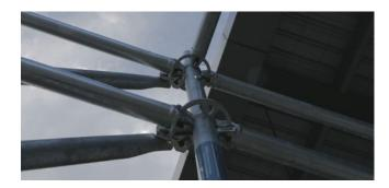
Load bearing braces allow users to build cantilevered bays out from one side, from behind a handrail; they are therefore never exposed to a fall. See more about this in our methodology.
