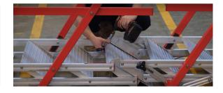
Using the hardware provided, secure the nuts and bolts together with an impact wrench, socket, and/or spanner
