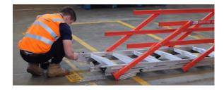
Align the two stairs on their sides, with the top batter stair's feet aligned to the bottom batter stair's top step
