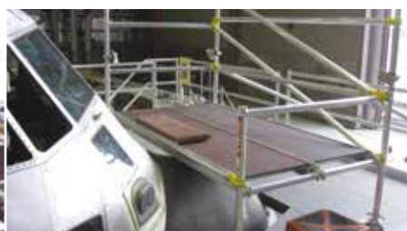
MOBILE SCAFFOLDING FOR WING PROTECTION DESIGNED TO AVOID USING HARNESSES AND LANYARDS
