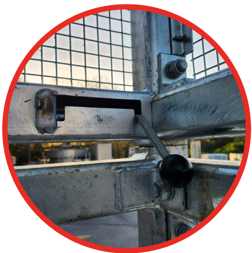
Sliding Pin Connection
