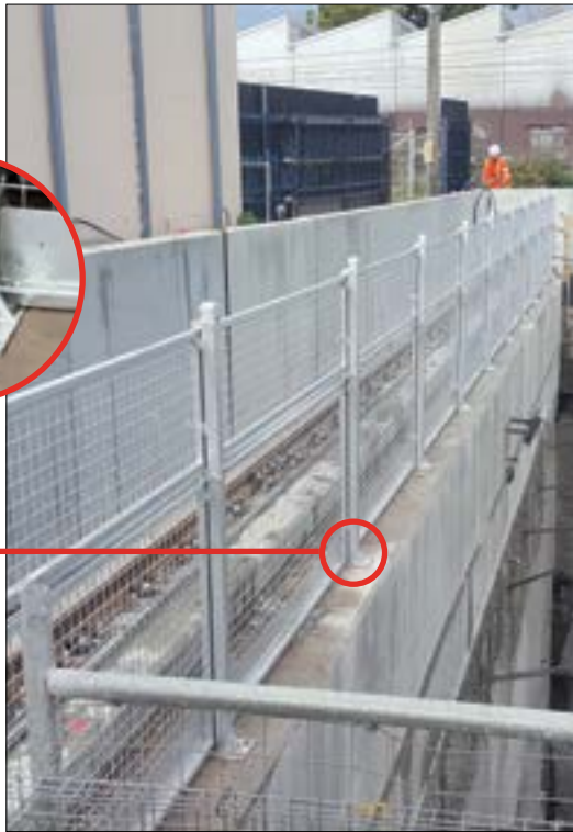
AdaptaPanel Slab Mount Post
