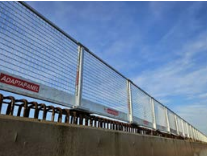
AdaptaPanel with Rebar
