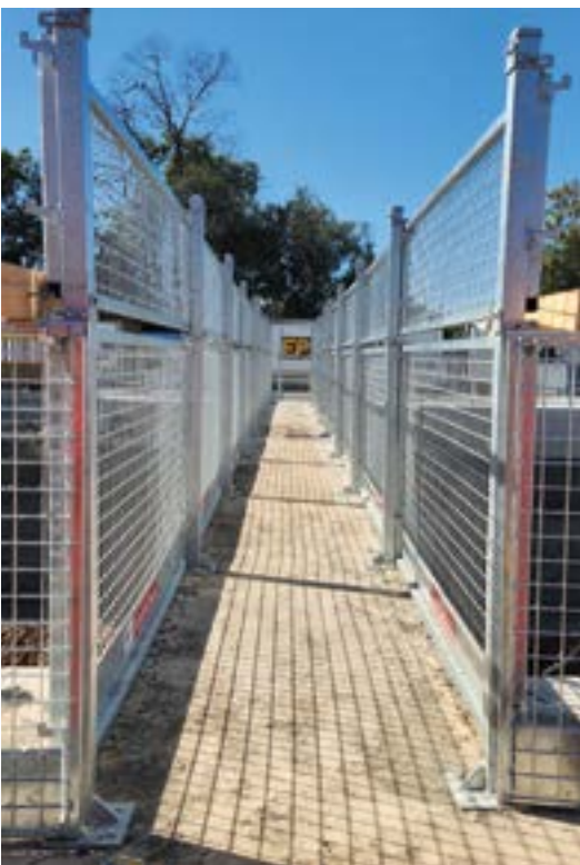
AdaptaPanel Slab Mount Post
