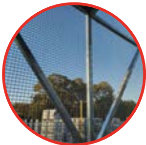
25mm x 25mm Mesh Encapsulation
