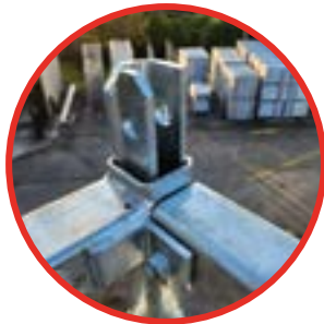
Certified Crane Lifting Points
