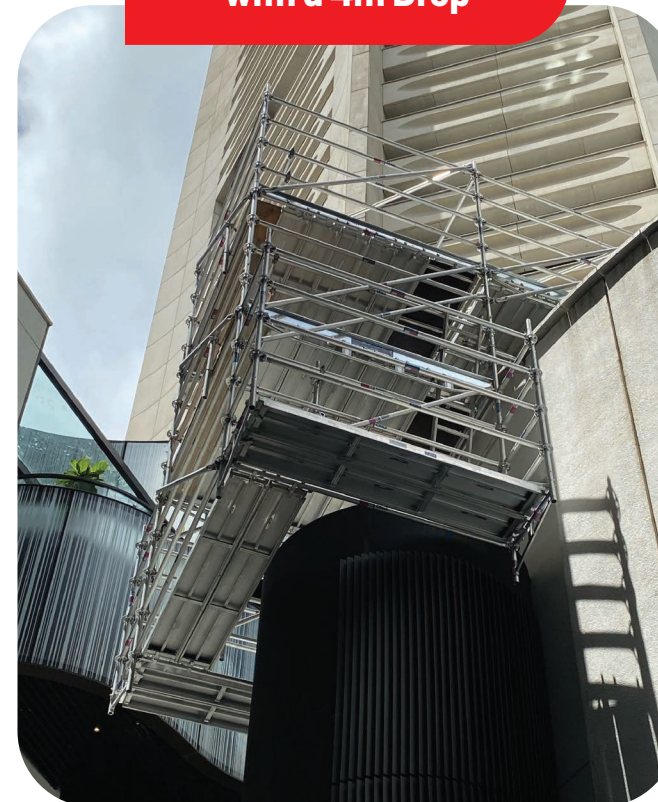
5m+ Cantilever with a 4m Drop
