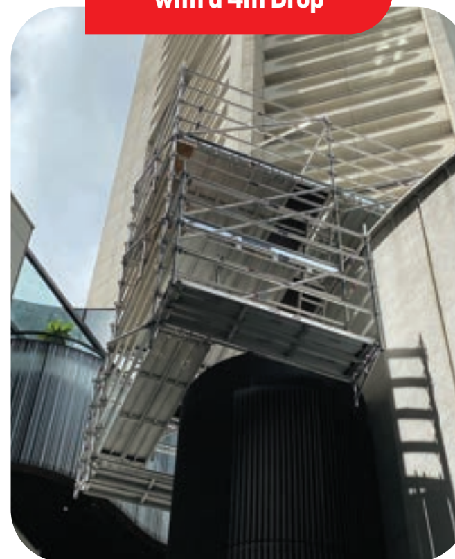
5m+ Cantilever with a 4m Drop
